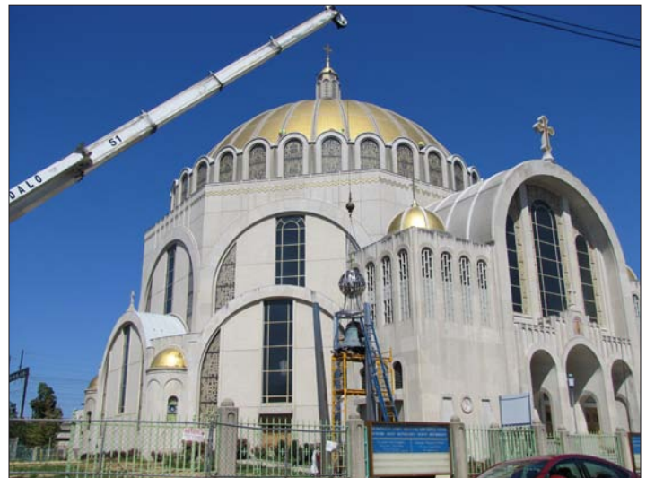
Workers install the top piece of the Bell Tower.
