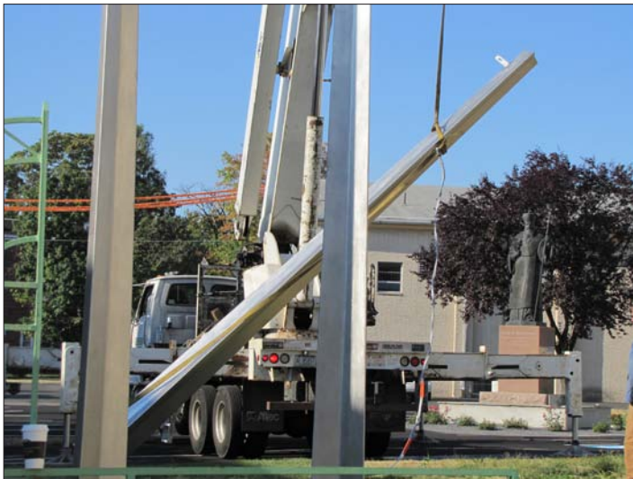
Workers install three pillars to support the Bell Tower.
