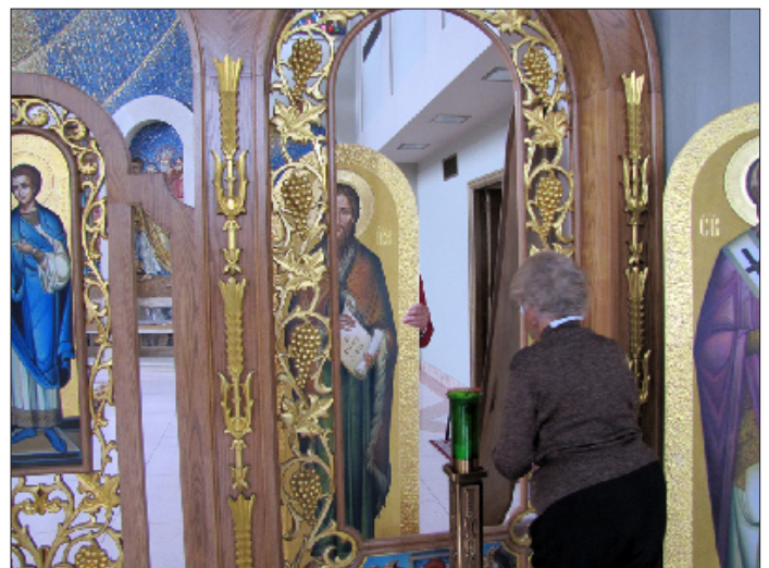
Christina Dochwat helps install the newly restored icon of St. John the Baptist to the iconostas.
