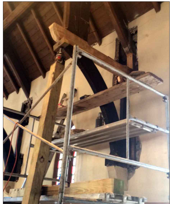
Original hammer beams of the 1950 Church being renovated and secured
